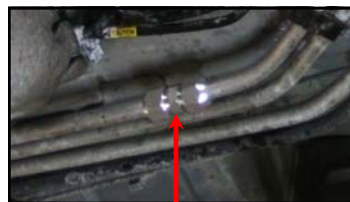
Repaired A/C Line w/S.U.R.&R. Union
